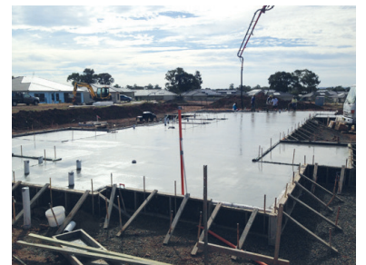
Quicker Finished Slab
