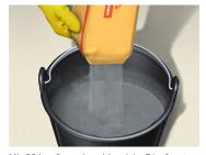
Mix 20 kg of powder with  $\sim 4.4 - 7$  L of water (depending on the desired consistency) in a suitable container.
