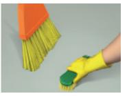
Surfaces must be sound, clean, free from oils, grease, and any loose or friable particles and other surface contaminants. Prepare the surface by appropriate means.
