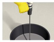
Mix with a low speed mixer, making sure to achieve a homogeneous consistency – at least 3 – 4 minutes.
